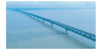
孟加拉帕德瑪大橋 Padma Multipurpose Bridge-Bangladesh
